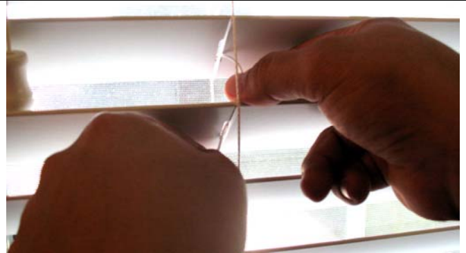
Step 4 – Re-thread the lift cord back down through the slats making sure to weave the lift cord through the ladder rungs from right to left.
