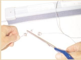
1. Remove shade from installation brackets. Unscrew joiner ball. Cut cords close to knot and washer.
